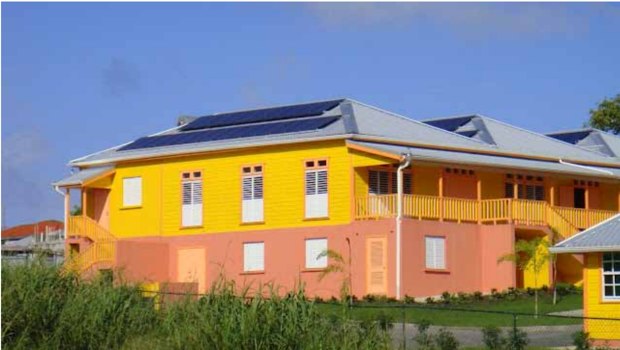
Scaling up efforts to integrate renewable technologies in public infrastructure – the new Sharon Primary School (Photo courtesy of the Natural Heritage Department)
