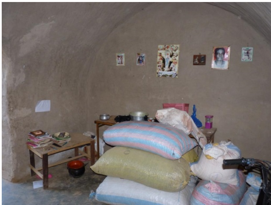
Figure 6: Adaptation measure: Roofing a house without wood in Dano 24
